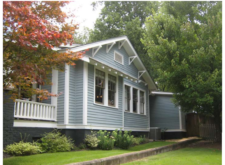
Right side of house from rear corner
