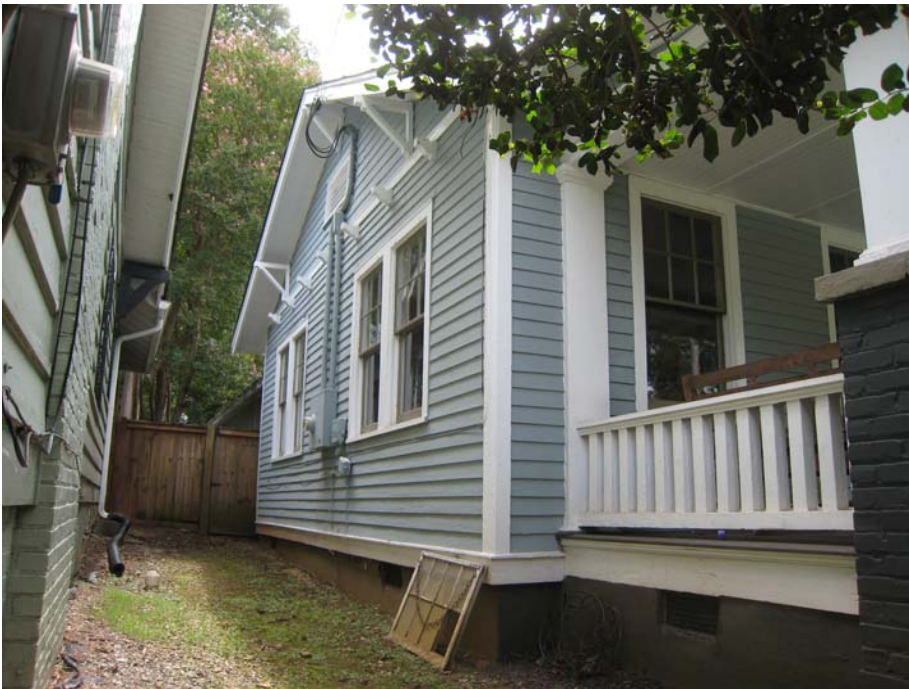
Left side of house from front corner
