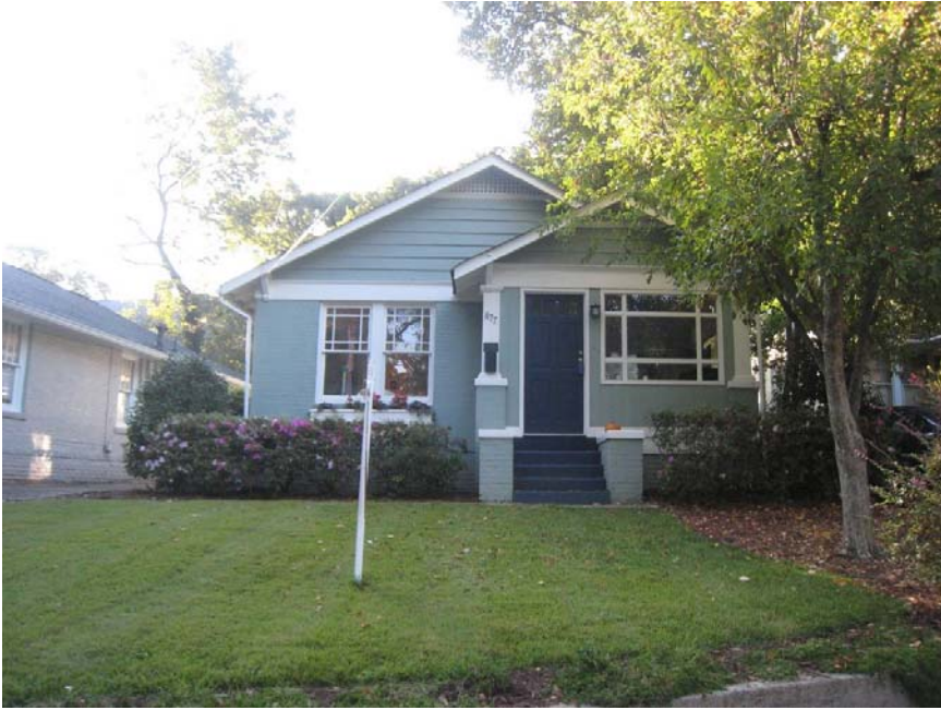
Front of house - existing porch to be reopened
