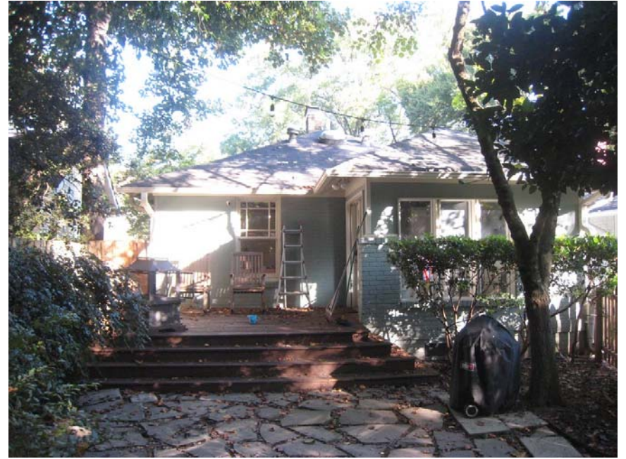
Rear of house - deck and patio to be removed
