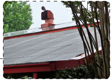
EXISTING 320 NORTH HIGHLAND - SKYLIGHT AT GABLE ROOF
