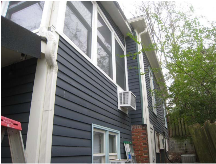
Left side of house from rear
