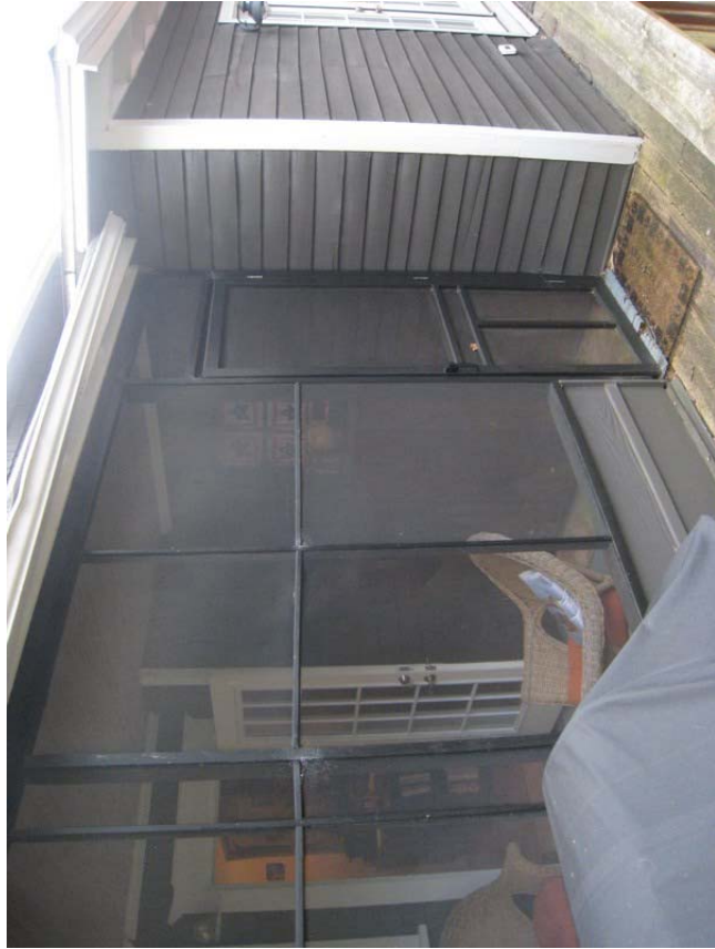
Non-historic screen porch and office addition to be removed
