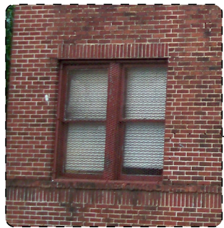
EXISTING 320 NORTH HIGHLAND - ORIGINAL DOUBLE-HUNG WINDOWS: SAME SIZE (36X72) & ALL EXIST. OPENINGS @ FRONT ARE SAME SIZE
