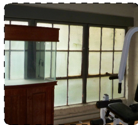
EXISTING WINDOWS - NEW TO MATCH EXISTING: STEEL OR STEEL "LOOK" WITH 3/3 LITE PATTERN
