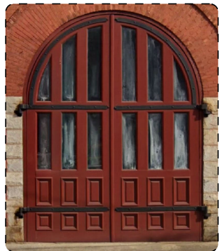
NEW CARRIAGE STYLE ENTRY DOOR; SIMILAR DOOR FOR REFERENCE AT 39 BOULEVARD NE - HISTORIC FIRE STATION CARRIAGE DOORS; NEW DOORS TO MIMIC THIS STYLE WHICH IS COMPATIBLE FOR THE TIME & DESIGN OF THE ORIGINAL BUILDING
