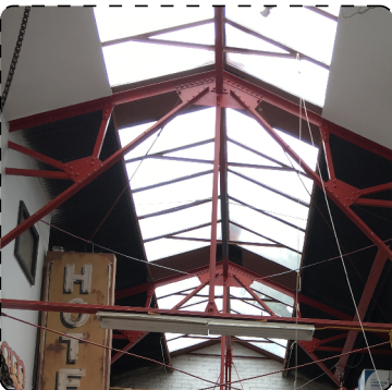
EXISTING 320 NORTH HIGHLAND - TRUSSES & SKYLIGHT AT GABLE ROOF
