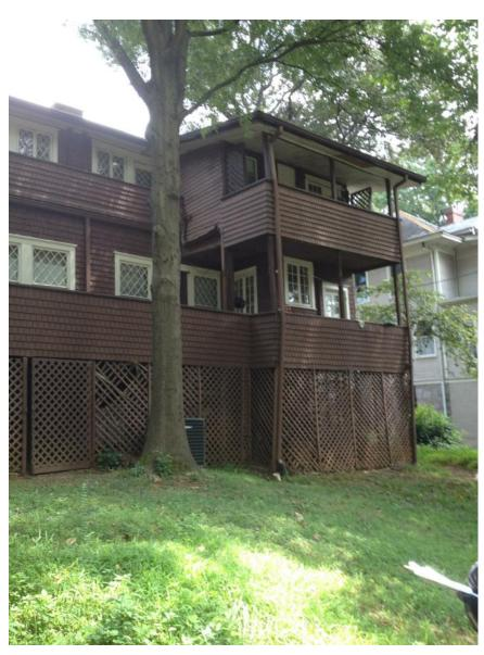
East wing at rear, note window differences in addition and haphazard drop down to fit porch under roof slope.
