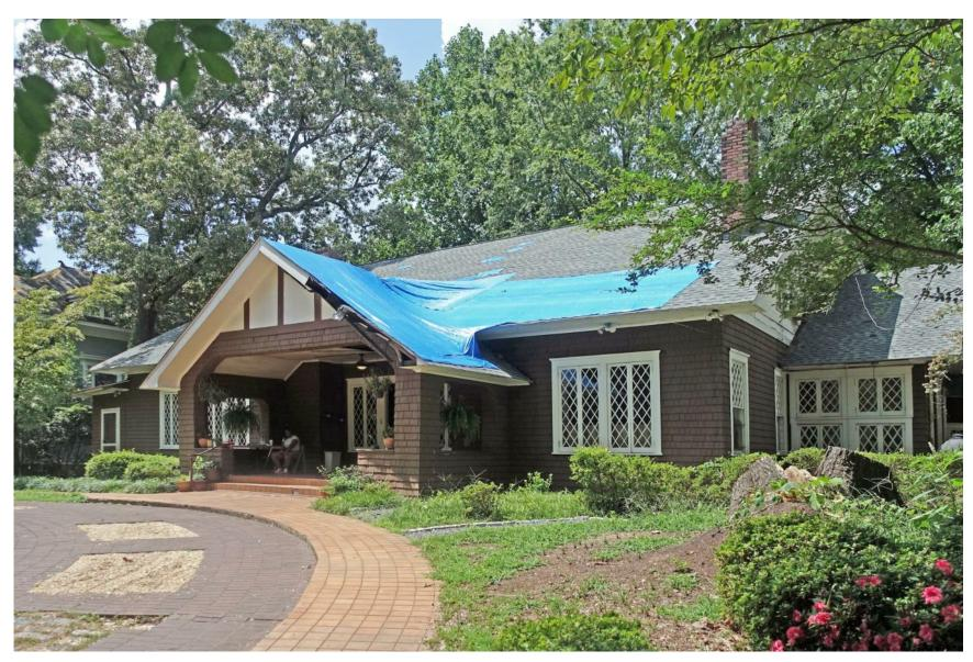
Current condition of front facade - note tree damage to front porch, right chimney, and main roof.
