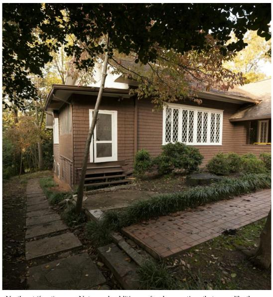
Northeast (front) corner. Note porch addition roof and proportions that are unlike the original construction.
