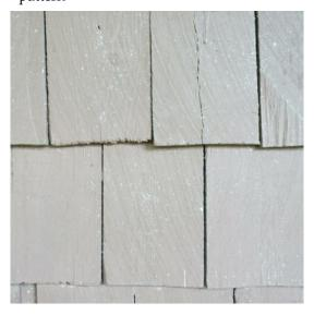
2 Cut shingles which appear to be much newer than the "original" shakes
