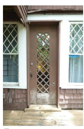
$\left< \begin{array}{c} Z \end{array} \right>$  Door type: probable 1970s door - note the thick muntins, stiles & rails.
