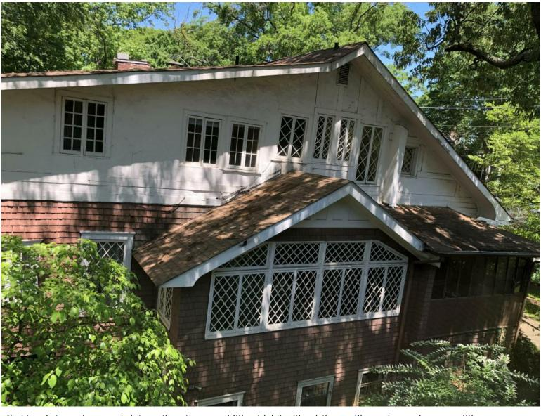
East facade from above - note intersection of corner addition (right) with existing roofline and curved eave condition - roofline to right not original. Note angled trim to left, likely indication of previous roofline.
