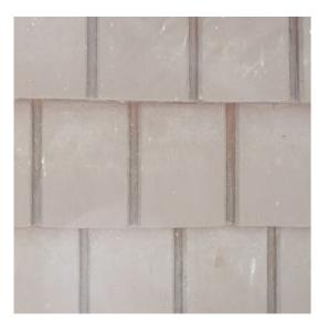
(3) T-III plywood cut and layered to resemble shingles - installed 1974-1994
